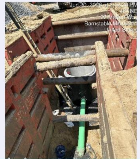
Sewer Manhole Installed on Marion Way
